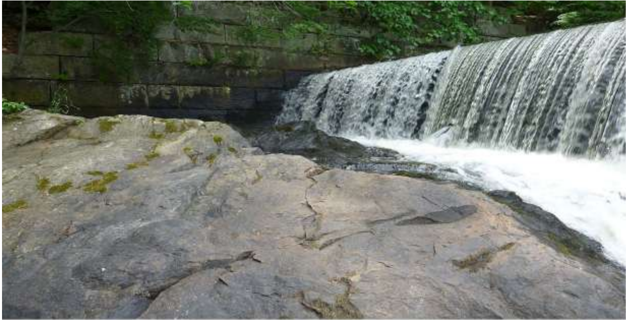
Figure A-2. South Side of Dam
