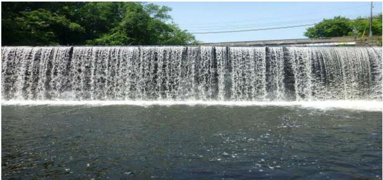
Figure A-1. Natick Pond Dam
