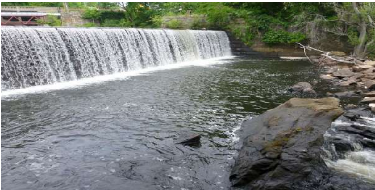
Figure A-3. North Side of Dam
